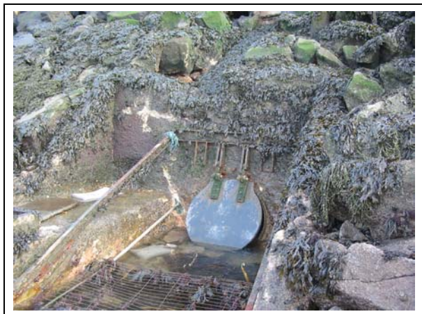
Photograph 1 - Flap valve on Seamill Pond Outlet
