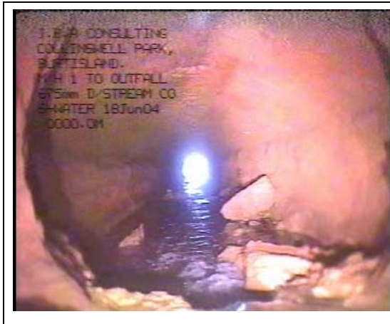
Photograph 2 – Railway Culvert Interior
